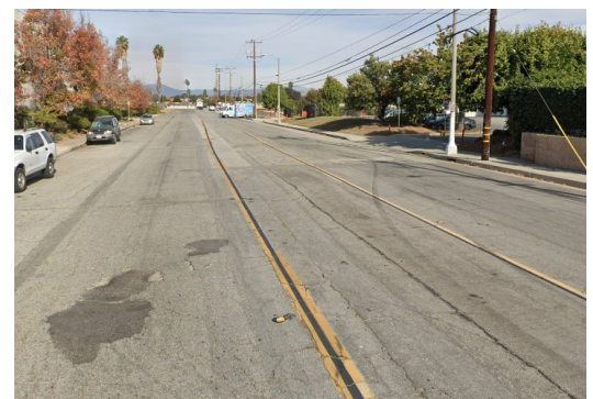
Marquardt Facing North
